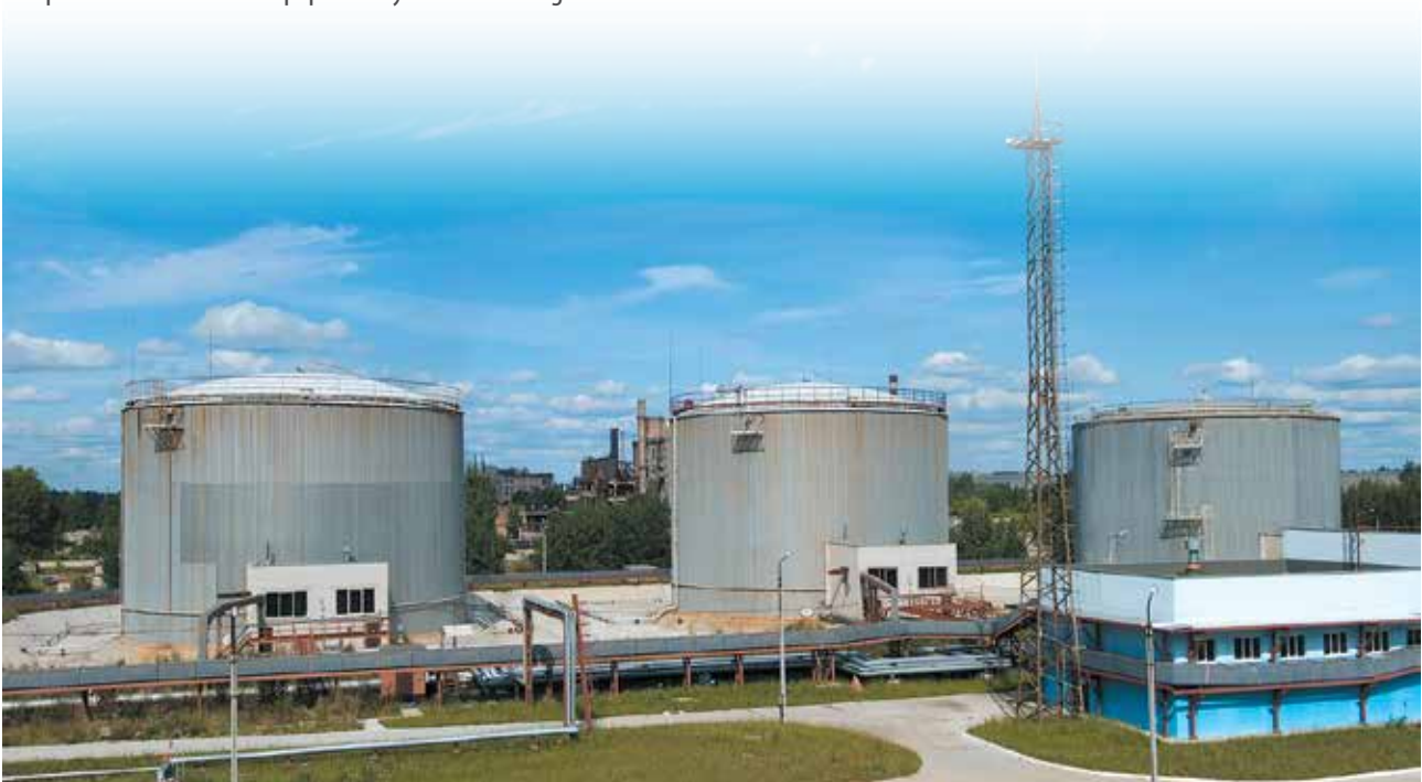
New fuel oil facility
