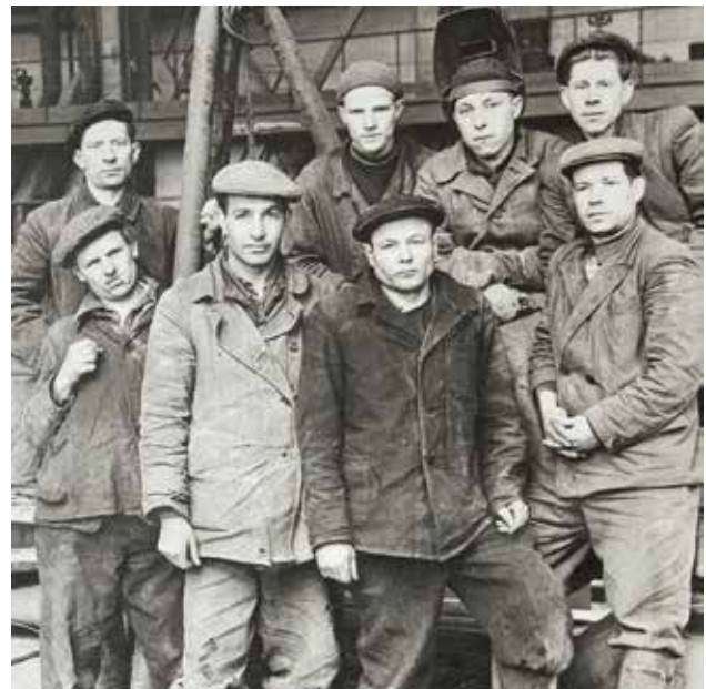
Lead crew of Ryazan branch of Central Electrical Installation business organisation under L.I. Chetverik during Boiler #1 installation. 1959
