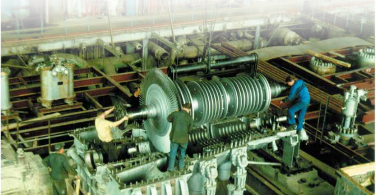
Installation of new Turbine Unit #1
