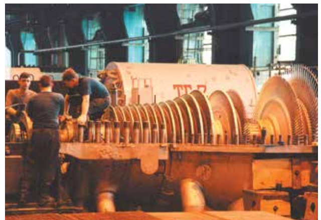
Installation of new Turbine #6
