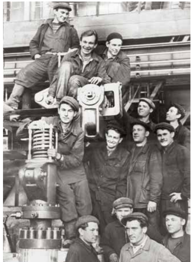
Installation crew of Ryazan branch of Central Electrical Installation business organisation on Steam Turbine #1. 1959
