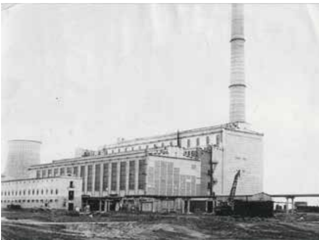
Construction of Novo-Ryazan CHP Plant. 1958
